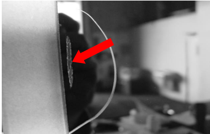
FIGURE 2-2: DEFECTS IN THE GLAZING
