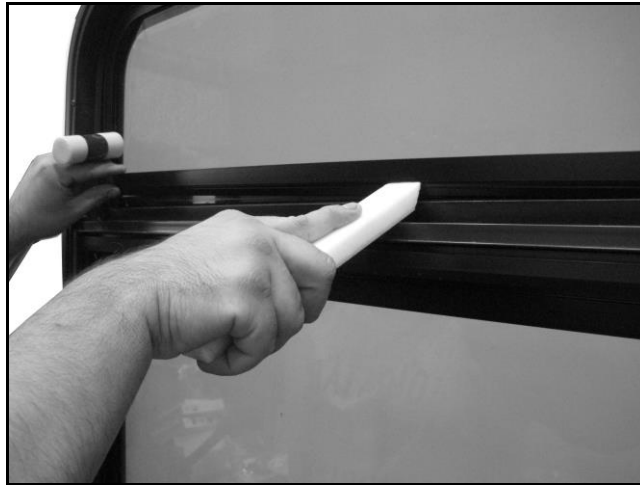
FIGURE 3-28: STANDARD FRAME HOPPER GLAZING REMOVAL
