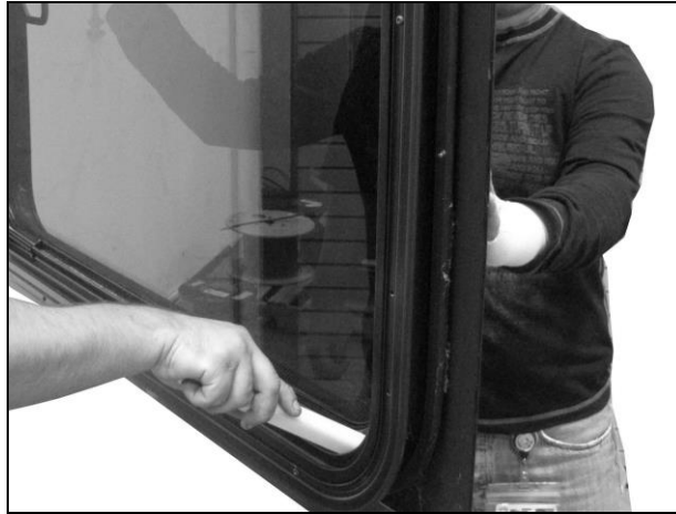
FIGURE 3-18. (EXAMPLE) TWO TECHNICIANS REMOVING HIDDEN FRAME CLIPS
