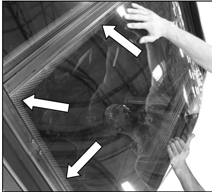
FIGURE 3-15. INSTALLING UPPER CORNERS
