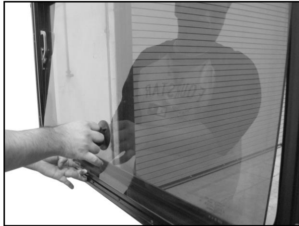
Figure 3-2. PULL STANDARD FRAME WINDOW GLASS GUARD USING SUCTION CUP
