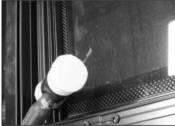
Figure 3-23. INSTALL HIDDEN FRAME CLIPS
